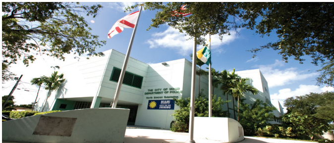
Miami Police North Station 1000 NW 62nd Street Telephone number (305) 795-2300
